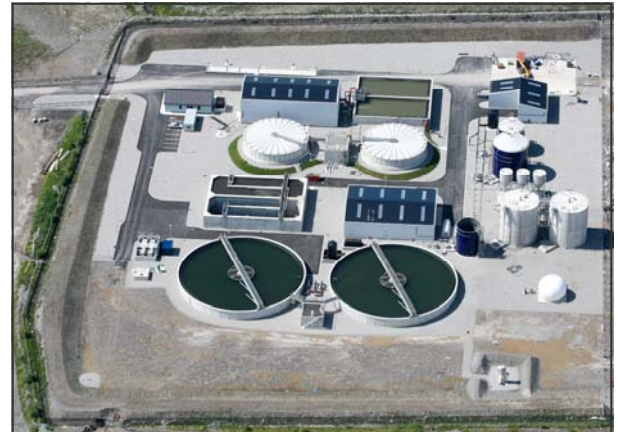
Aerial view of the new Sligo Wastewater treatment Plant at Finisklin
